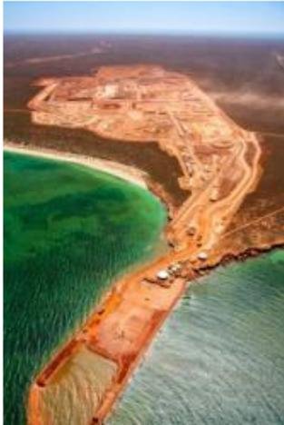
The Marine Offloading Facility (MOF) foundations begin to extend from the gas plant footprint. The MOF will enable the offloading of materials required for the Gorgon Project.
